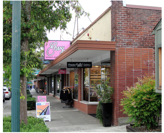
3811-13 N. 26th, showing 1962 facade addition, 2019
