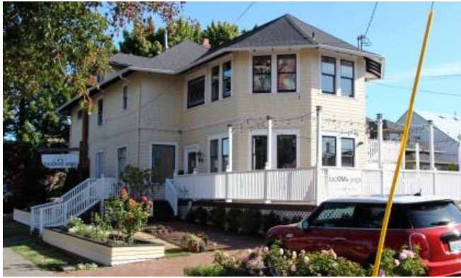
2717 N. Proctor, southwest rear facade, 2019
