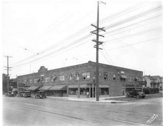
Gamble Building, 1930 (Boland, B22748)
