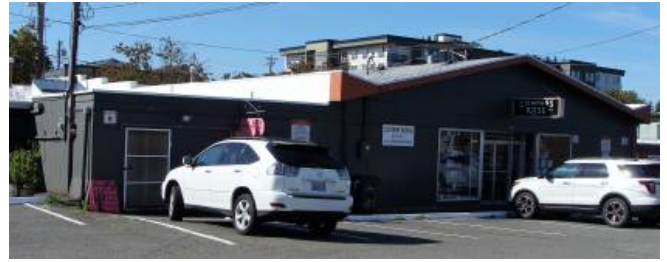
3815 N. 26th, rear facade, 2019
