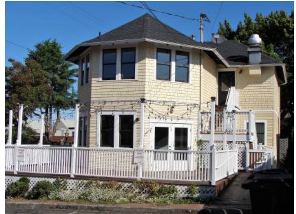
2717 N. Proctor, southeast rear facade, 2019
