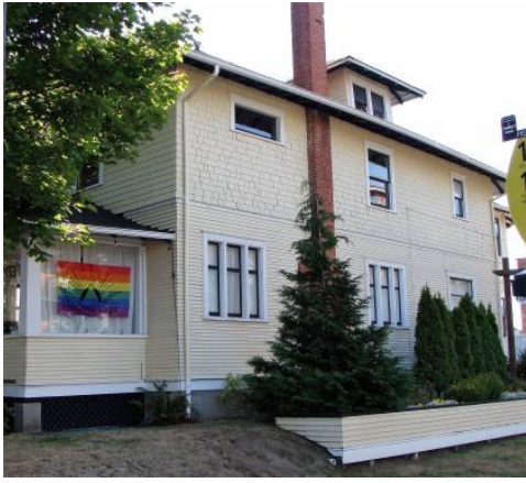
2717 N. Proctor, west facade, 2019
