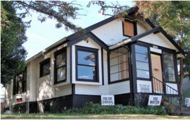
3810 N. 27th St., north & east facades, 2019
