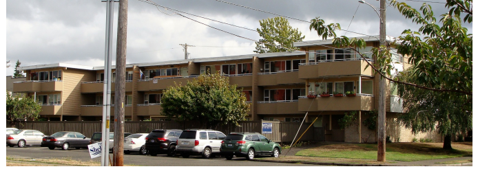
Mason Manor, north facade, 2019
